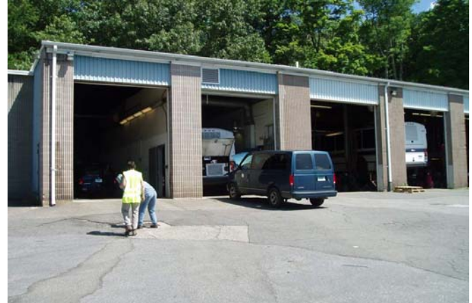
Figure 2. Motorpool parking lot (top) and existing external
