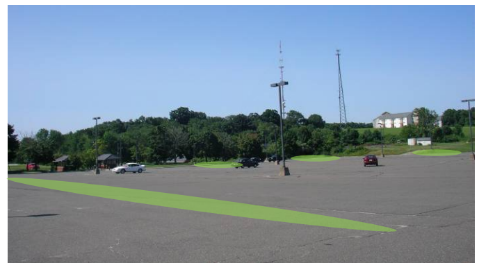
Figure 2. Approximate location of proposed bioretention cells in parking lot. Restriping of lot will be required around landscape island bioretention to alter current traffic flow patterns. Loss of only four or five spaces anticipated.
