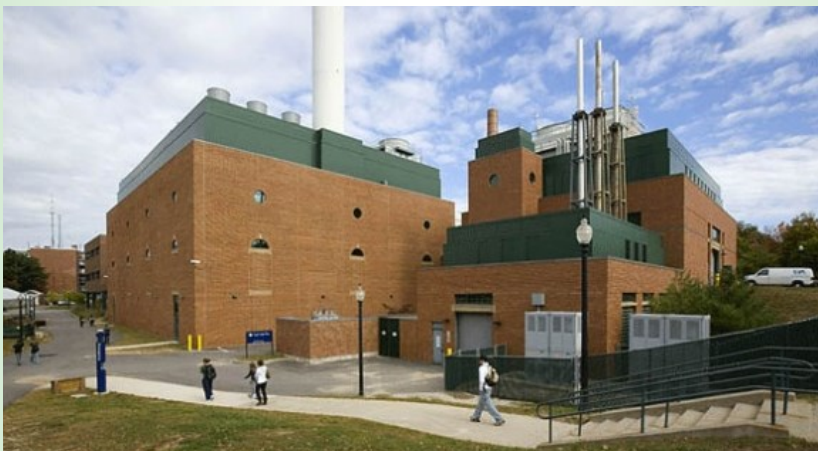
Central Utility Plant and Cogeneration Plant at UConn Storrs Campus
